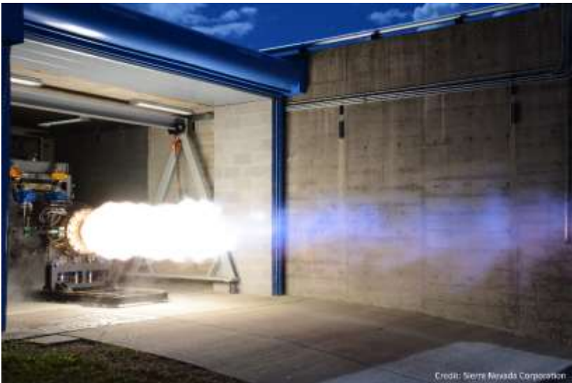
Figure 11. Rocket Test Facility
